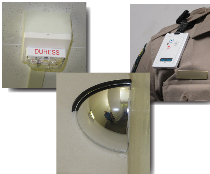
Examples of corrections (left to right): blinking alarm light, bubble mirror to see blind areas, personal alarm
